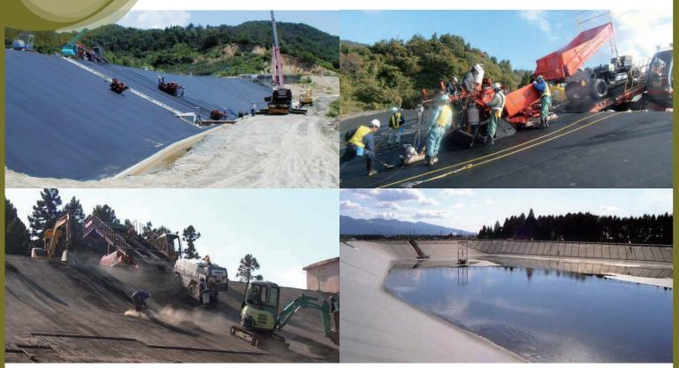
Creates a surface shielding membrane using a watertight asphalt mixture for treatment facilities and reservoirs.
